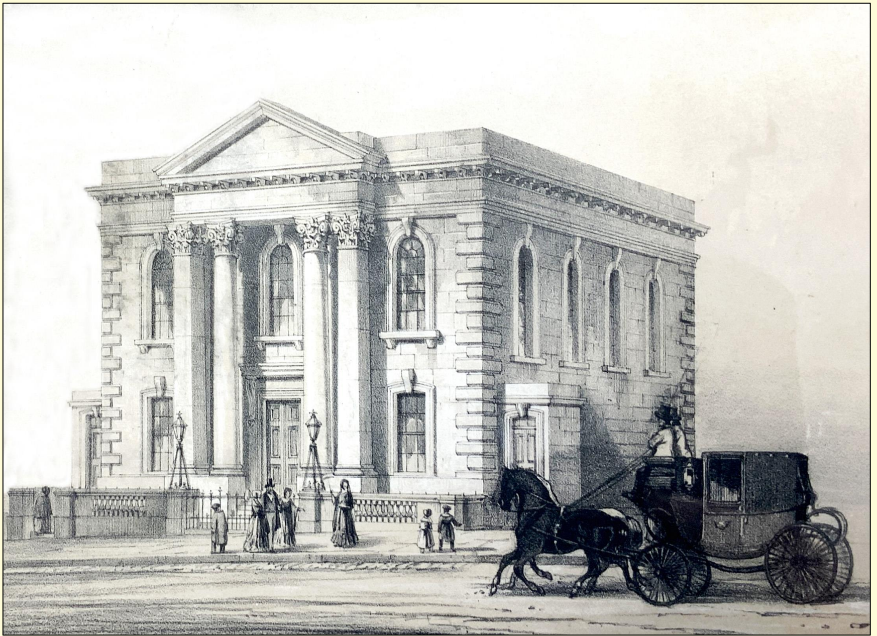
Moravian Chapel, Charlotte Street – James Wilson Architect built in 1845
