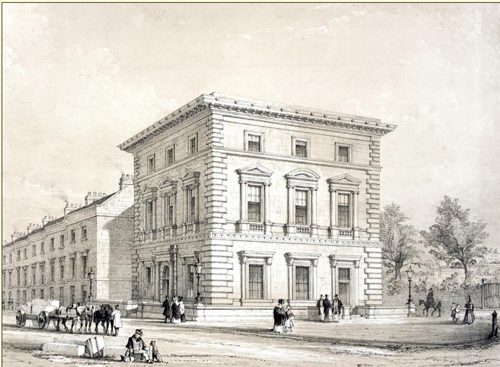
Bath Savings Bank designed by George Alexander. Built in 1841
