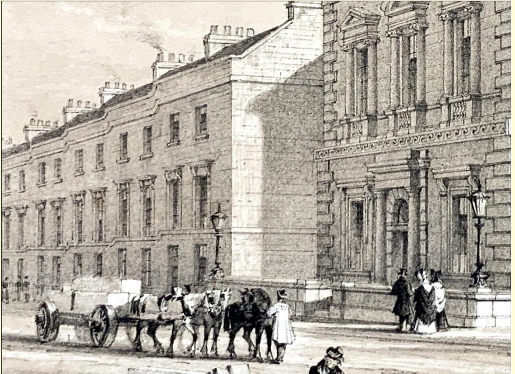
Charlotte Street Terrace designed by George Phillips Manners in 1839.
